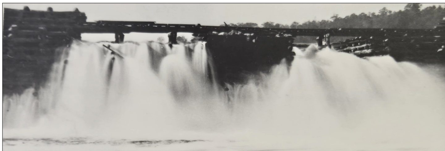
1860 log dam on Indian Lake
