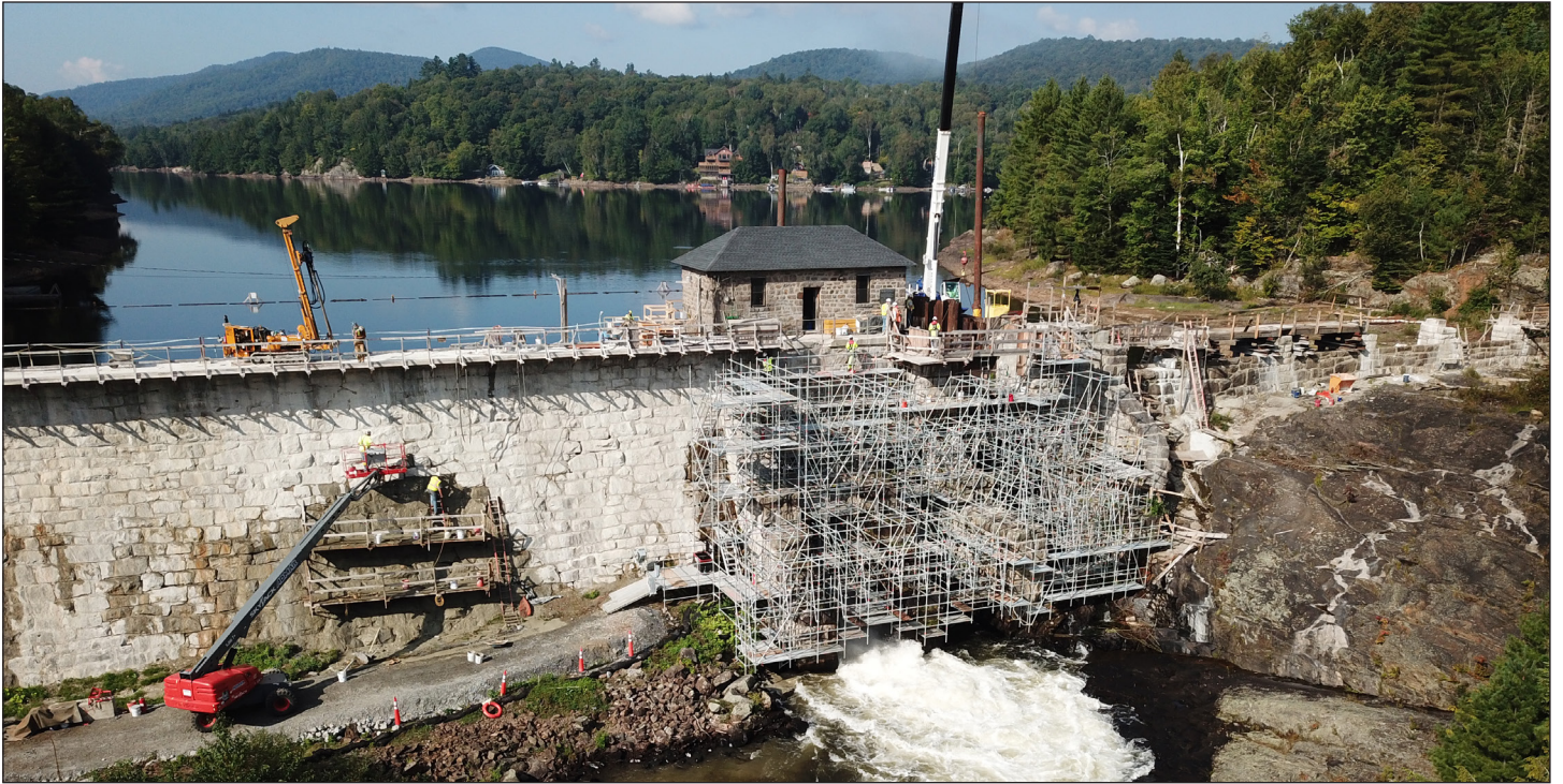
Indian Lake dam rehabilitation work summer of 2024. Photo courtesy of HRBRD and Colliers Engineering and Design.
